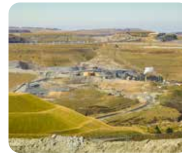
↑ A rehabilitated waste rock stack and the processing plant at our Macraes Operation, New Zealand
