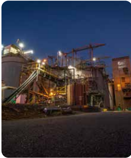
↑ Waihi Operation's processing plant, New Zealand
