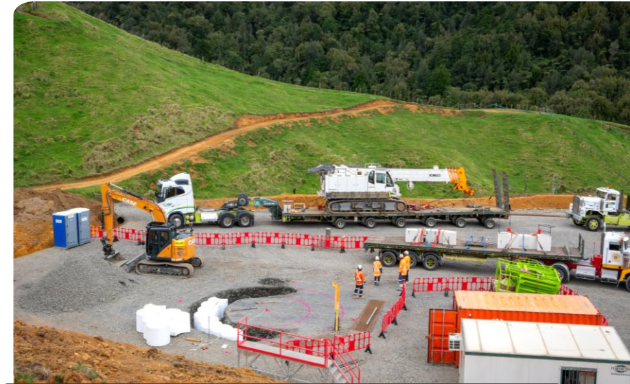
Vent shaft 1 construction – September 2026
