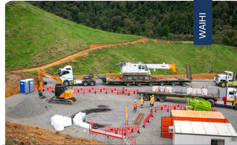
Vent shaft 1 construction – September 2026
