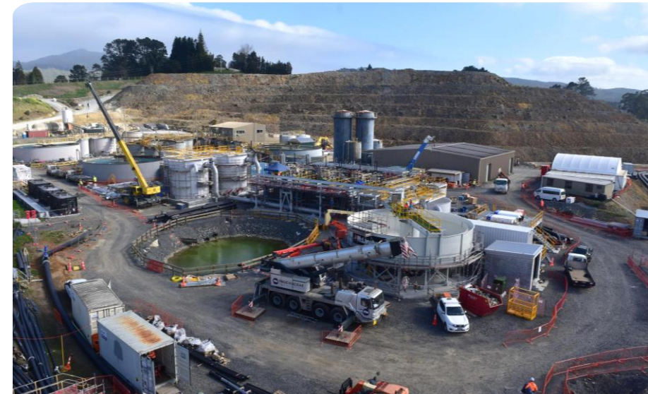
Water treatment plant – September 2026
