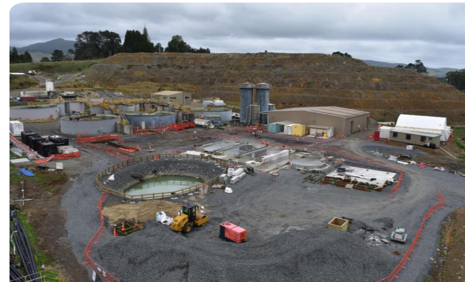
Water treatment plant – March 2026
