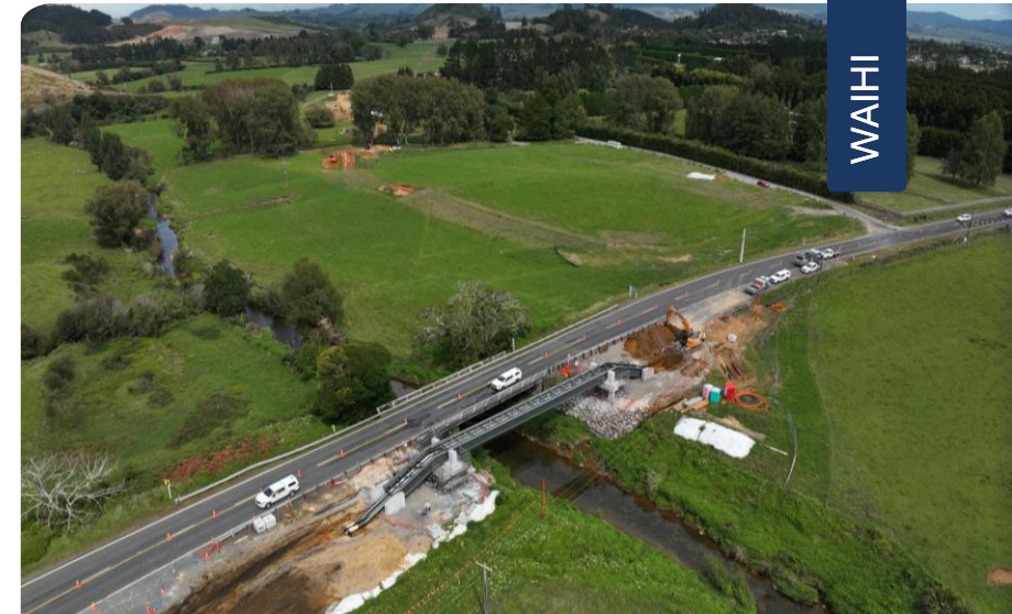
Services trench – March 2026
